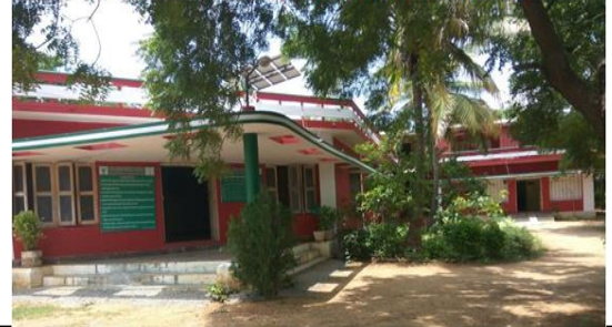
Administrative Cum Office Building
