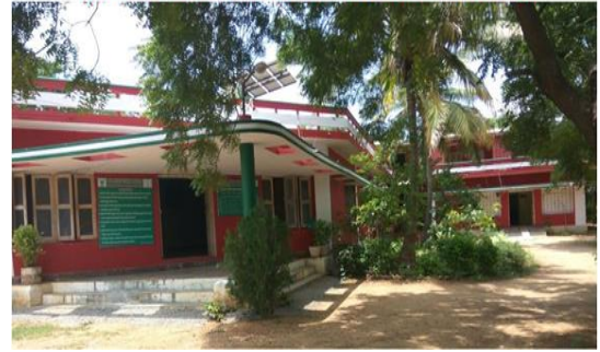
Administrative Cum Office Building
